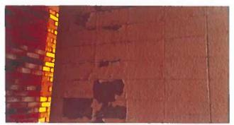
Spalling was noted on the exterior concrete block texture.
